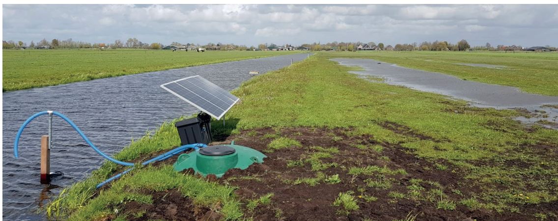
Foto: Waterinfiltratiesysteem (WIS)
